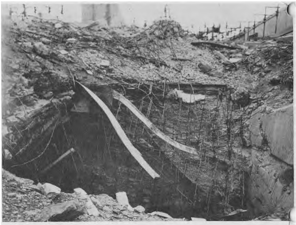
BREST—U-BOAT PENS. A 12,000 lb. bomb crater through 19'6" reinforced concrete U-boat shelter roof.
