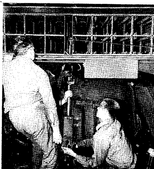
Figure 47—Screwing Elevating Strut Into Block on Launcher
