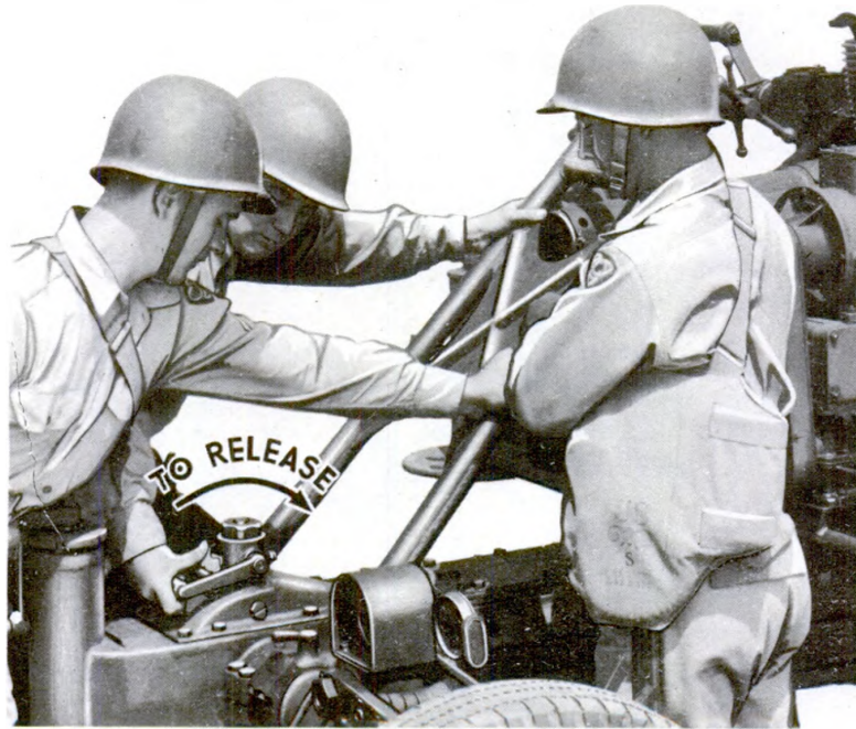
Figure 84 – Unlocking Rear Chassis Compensating Spring Lock
