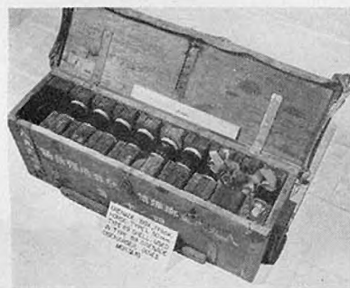
Figure 53.—Two views of packing box for Model 89 (1929) 50-mm shells, showing method of packing individual shells (40 rounds without fuzes).
