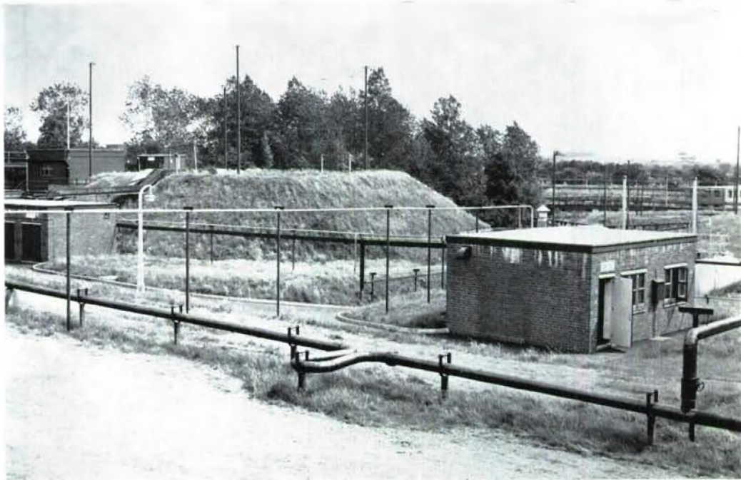
Fig. 21 External view of control room for Biazzi plant
