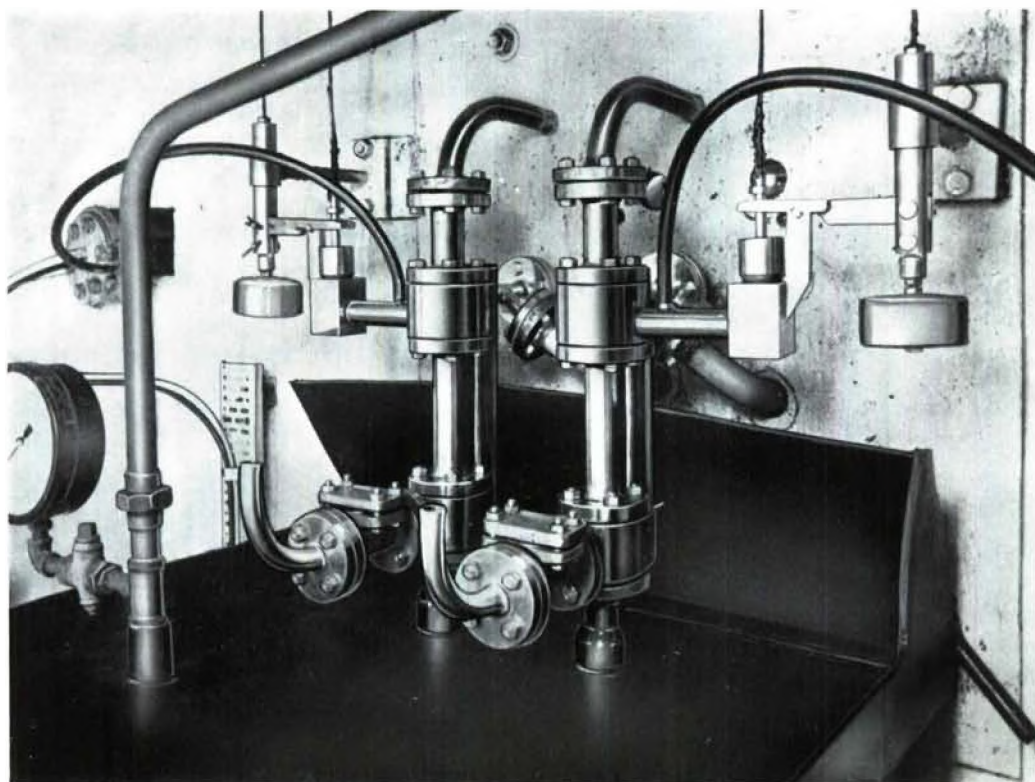
Fig. 23 Two injectors for dual stream nitration of glycerine
