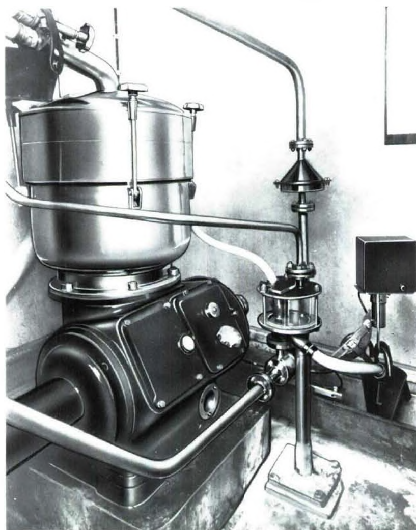
Fig. 24 Centrifuge for separating nitroglycerine from refuse acid
