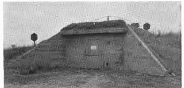
FIGURE 10. Large concrete magazine at Blossom Point.
