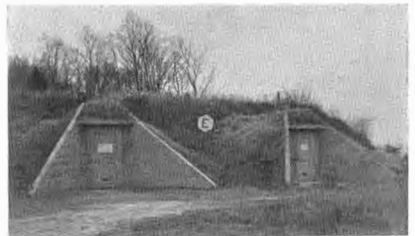
FIGURE 9. Smaller concrete magazines at Blossom Point.
