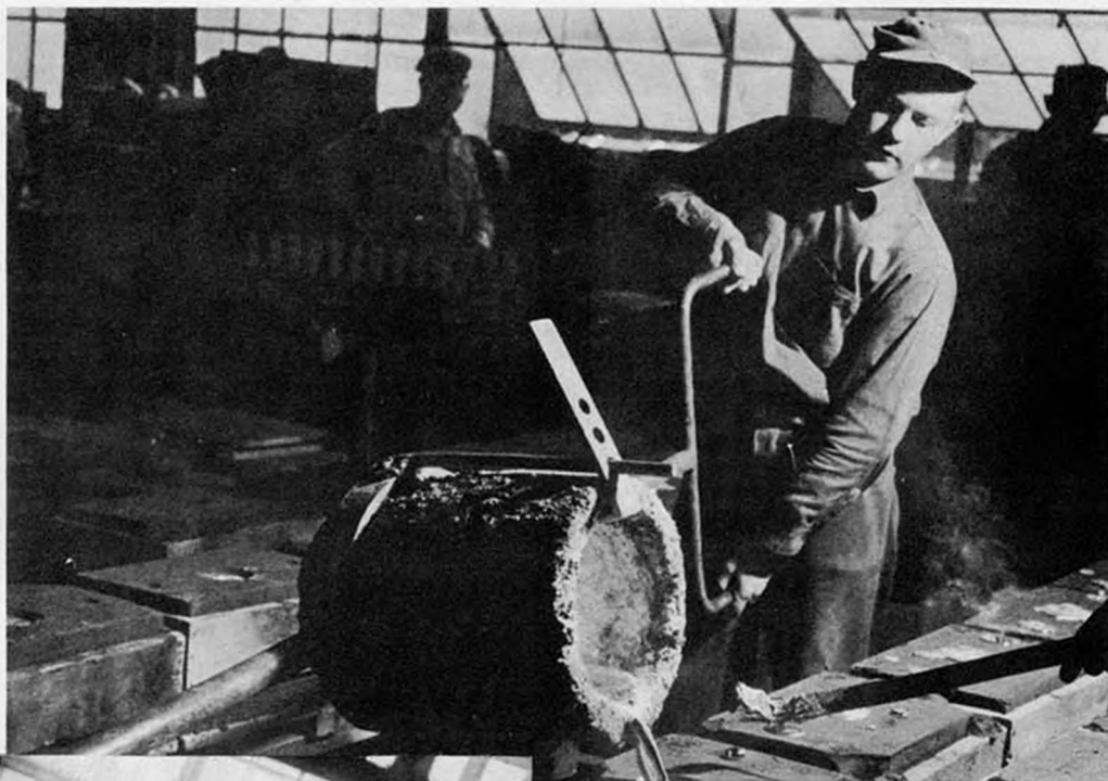
Pouring the molten aluminum alloy into the moulds. The Bausch and Lomb Foundry is on a three-shift basis with a 24-hour working schedule.
