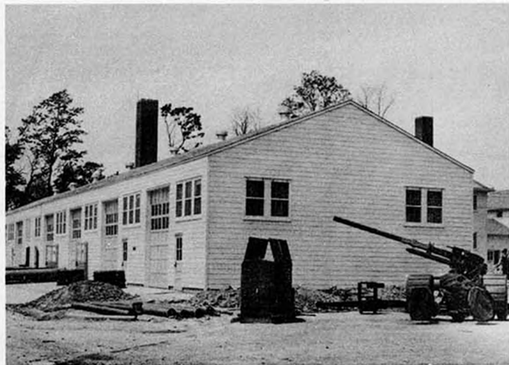
ANTI-AIRCRAFT FIRE CONTROL BUILDING
