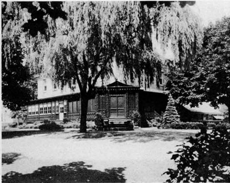
Commanding Officer's Quarters, constructed 1823
