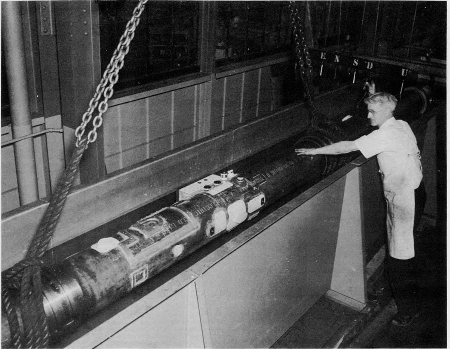
Above: Range Finders are filled with compressed gas and immersed in water to reveal leaks. Below at left: Skilled hands prepare a Range Finder
