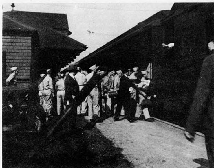
The first Bomb Disposal unit entraining for field duty.
