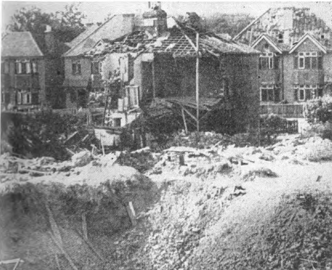
Figure 38. Bomb Explosion Near Building.
