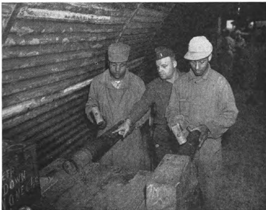
Figure 21. Removing Dents from Shell Cases.
