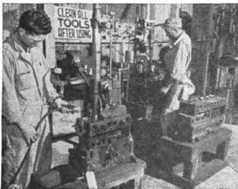
Cylinder Reboring and Honing.
