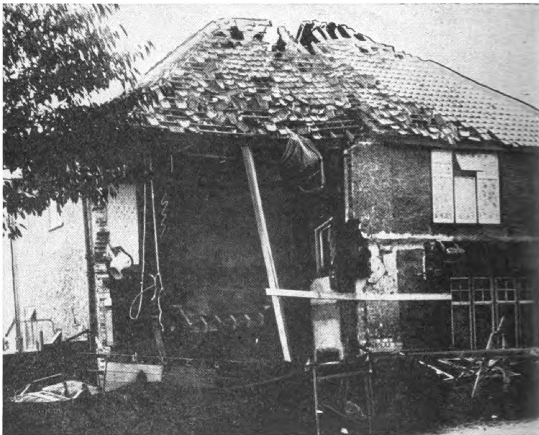
Figure 41. Damage Due to an Unexploded 250 Kg. German Bomb.
