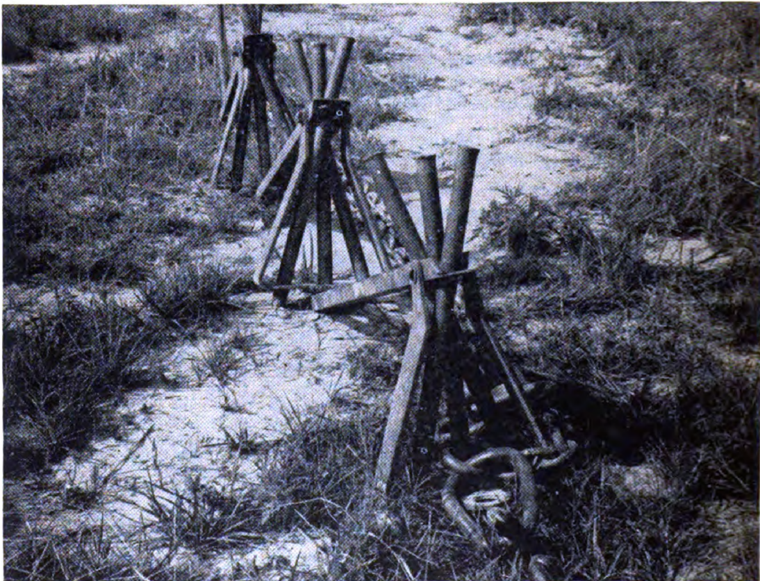
Figure 51. Holmes Ground Anchor.
