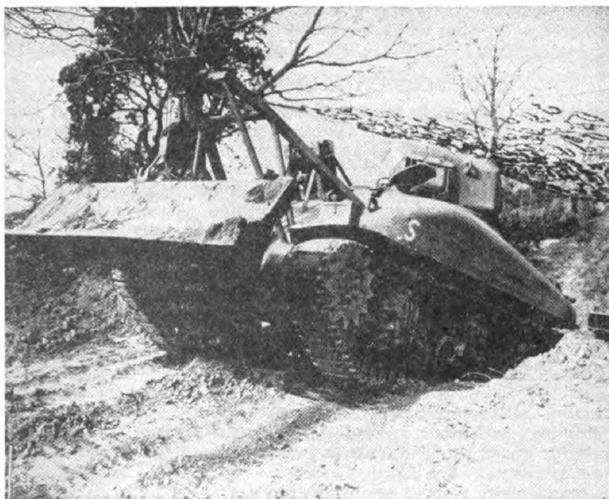
Figure 18. Bulldozer Blade Mounted on Medium Tank M4.
