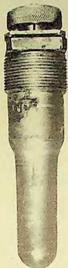
Fig. 181 Type 3 Electric Gauge.
