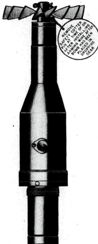
Figure 17.—Tail Fuze AN-Mk 228
