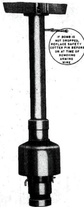
Figure 31.—Tail Hydrostatic Fuze Mk 240 Mod 0
