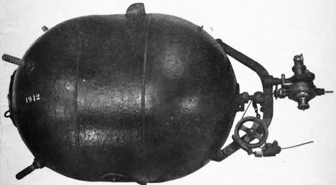
Figure 2—JA mine without anchor.
