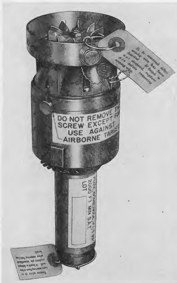
Figure 5—Ring Type VT Bomb Nose Fuze, Model T93.
