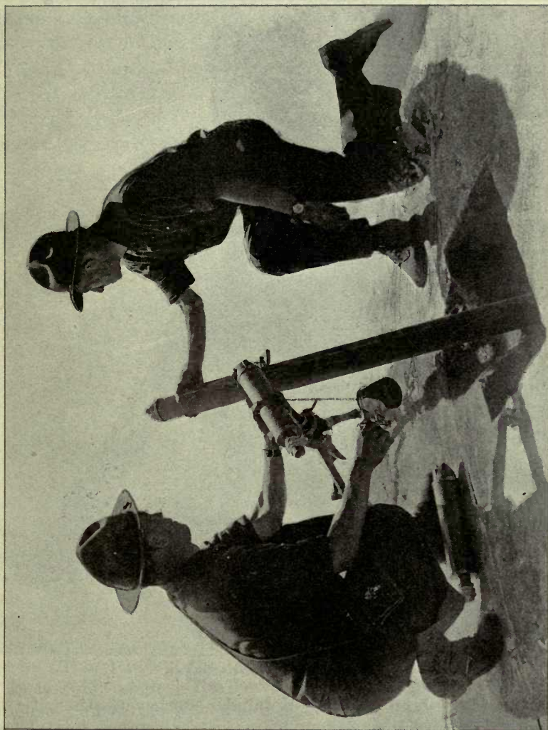
3-INCH STOKES TRENCH MORTAR, MARK I, SHOWING MORTAR IN ACTION.
