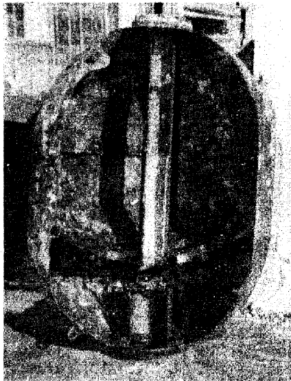
Fig. 3. Sectionalized View of Type 92 Mine Case
