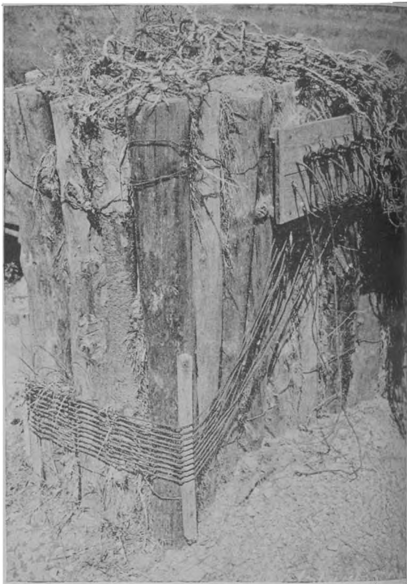
The central switchboard for the fougasse flame throwers shown in the preceding photographs.
