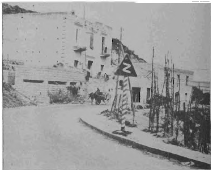
This pillbox was built to cover a road bend in Baia, south of Rome. The blocks with which it is faced blend with the wall of the house behind it.
