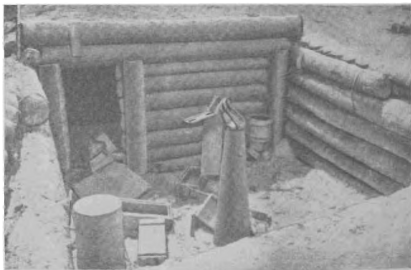
Figure 12.—Emplacement for Japanese Single-mount 13-mm Machine Gun.
