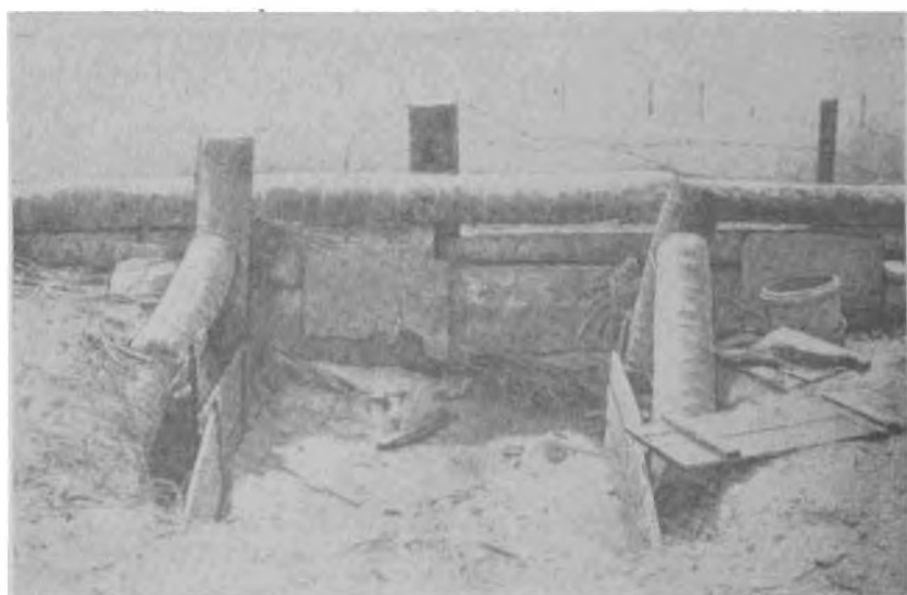
Figure 6.—Japanese Open-type Rifle or Light Machine-gun Emplacement.
