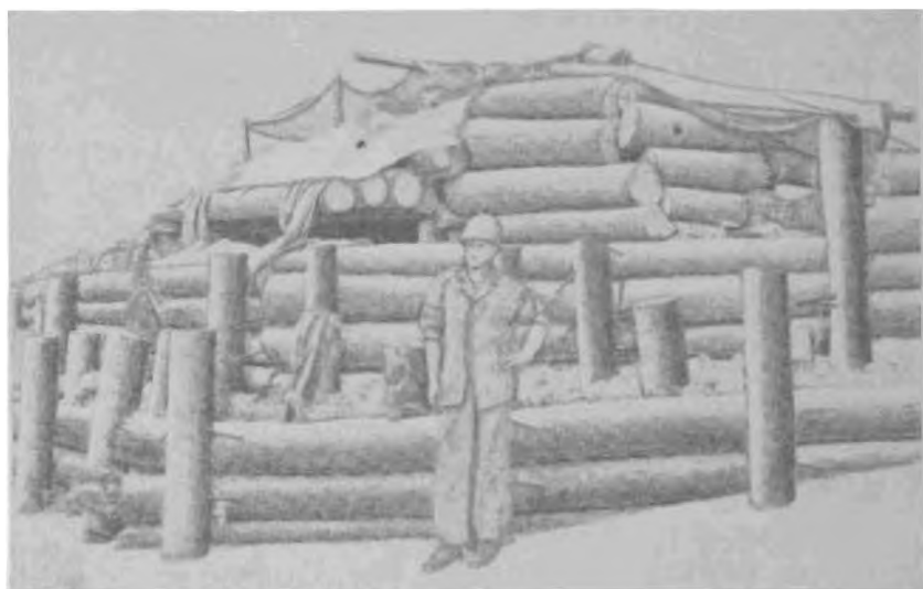
Figure 9.—Japanese Heavy Machine-gun Emplacement (as an integral part of a beach barricade).
