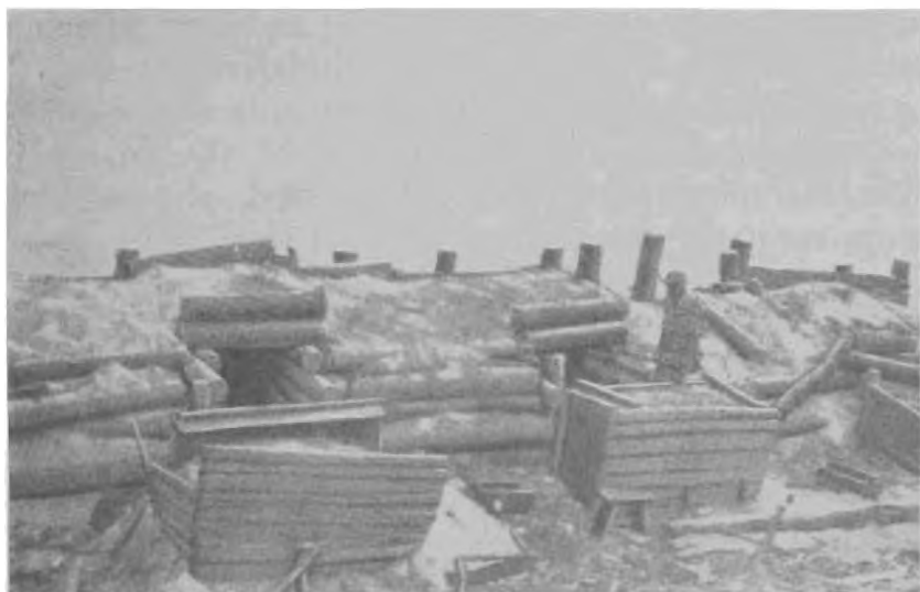
Figure 5.—Rear View of Japanese Rifle or Light Machine-gun Emplacements (showing type of construction, blast walls protecting entrances, and the spacing between each pit).
