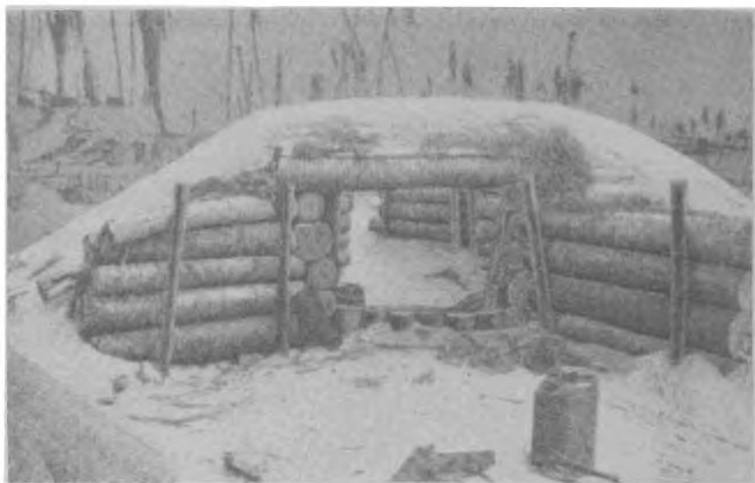
Figure 14.—Emplacement for Japanese Field Gun.
