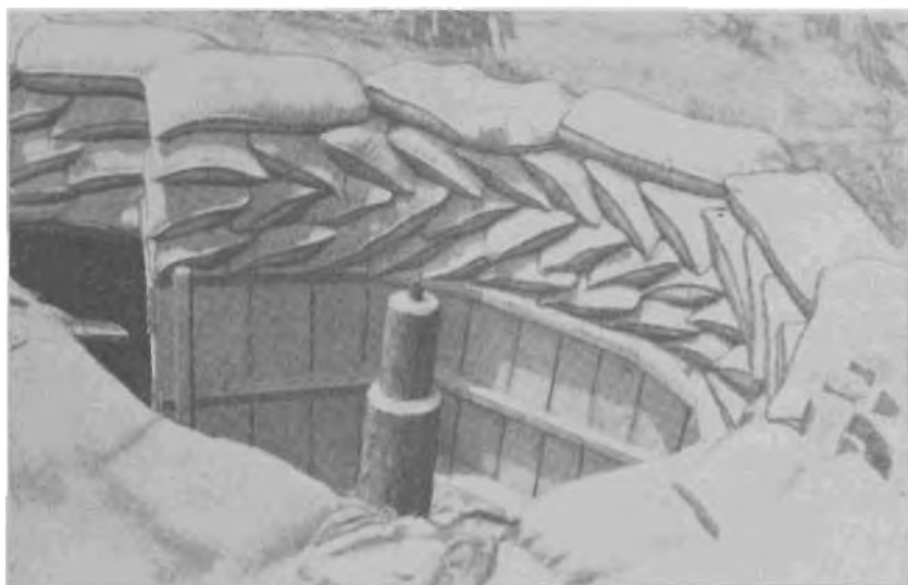
Figure 11.—Japanese Open-type Heavy Machine-gun Emplacement (primarily for antiaircraft).
