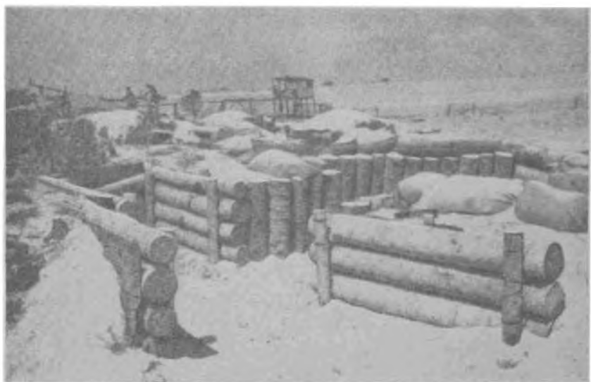
Figure 15.—Open Emplacement for Japanese Field Gun (probably for 70-mm battalion gun).
