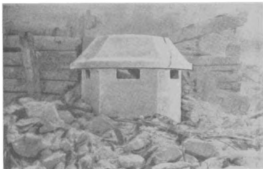
Figure 7.—Japanese Reinforced-concrete Emplacement (provides both frontal and flanking fire for light machine guns).
