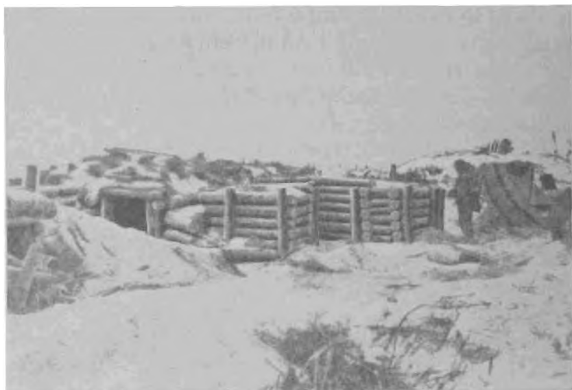
Figure 10.—Rear View of Japanese Heavy Machine-gun Emplacement (showing ammunition storage room in rear; entrance; and rifle or light machine-gun emplacement to left).
