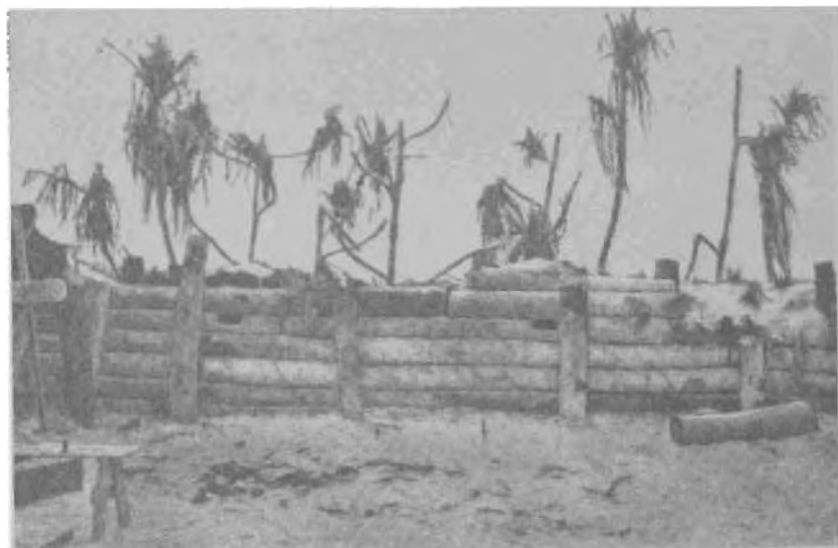
Figure 4.—Japanese Beach Barricade (with built-in rifle or light machine-gun emplacements).
