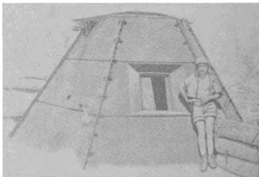
Figure 16.—Japanese Steel-pillbox Command Post (side view showing firing port).
