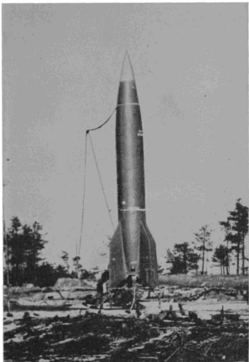
A significant feature of a V-2-type guided missile is the simplicity of its launching site. In respect to mobility and use of a rapidly-prepared and suitably concealed position, these missiles resemble field artillery.
