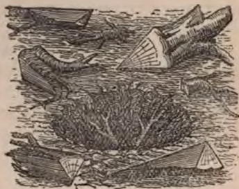
FIG. 57.—SAME STUMP AFTER BLASTING.
