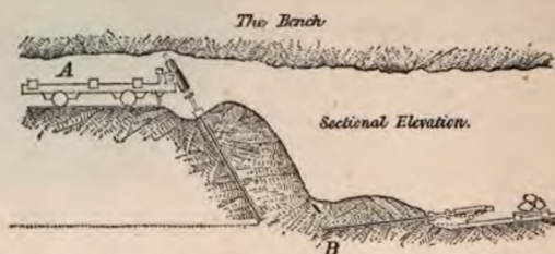
FIG. 72.—SECTION OF BENCH-WORK AT MUSCONETCONG TUNNEL.
