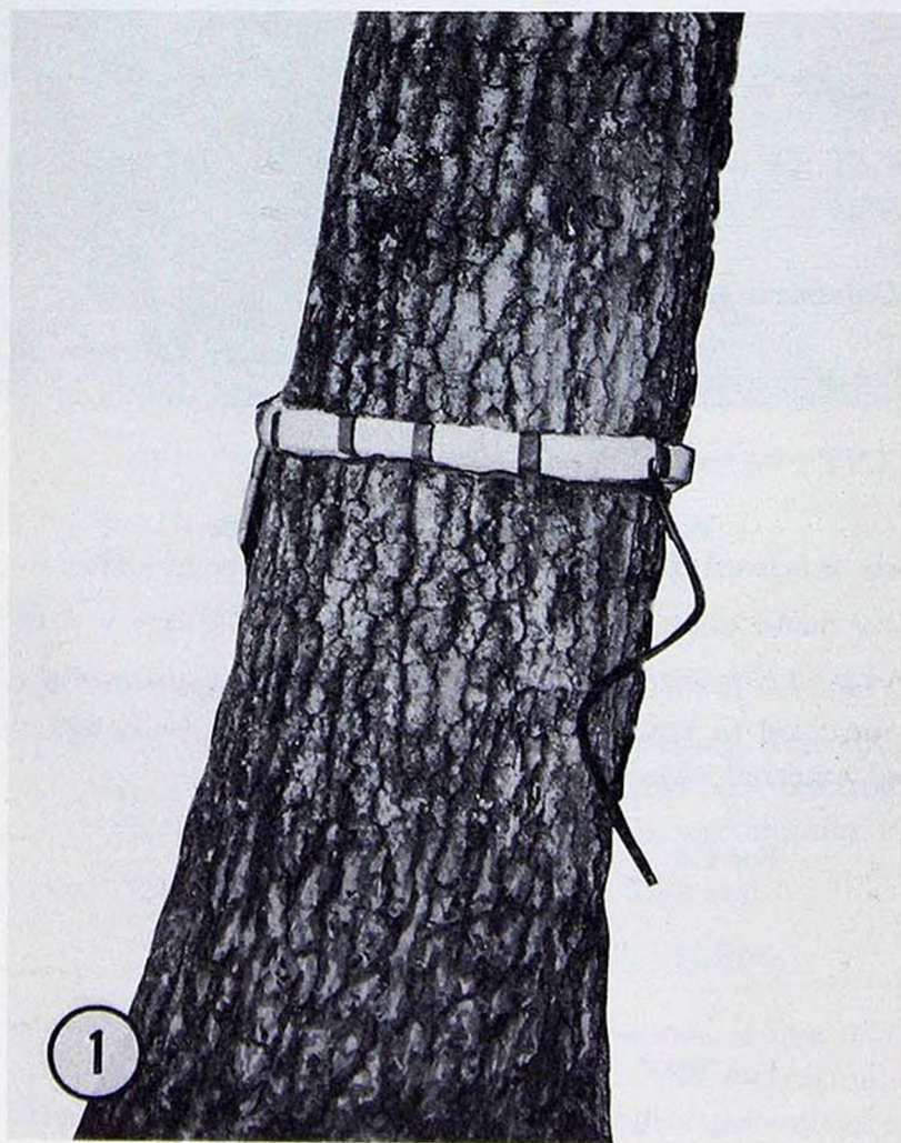
1 Composition C4 charge completely encircling tree.
