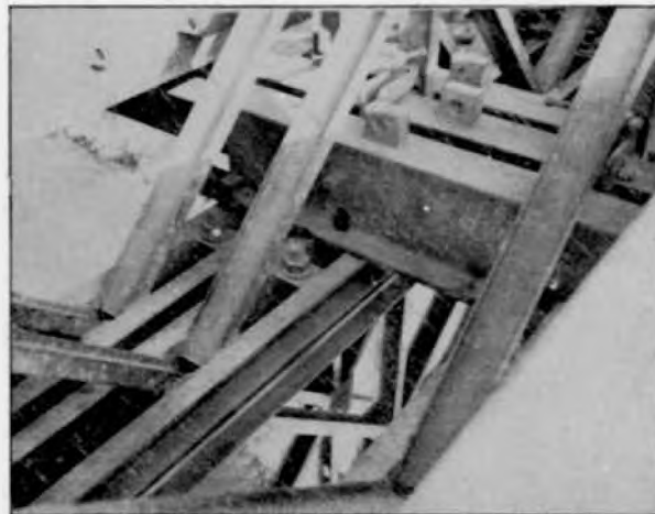
TOP VIEW REINFORCING CENTER TRUSS PLATE 9
