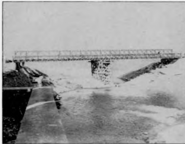
FIG. 1 BRIDGE PRIOR TO REINFORCING
