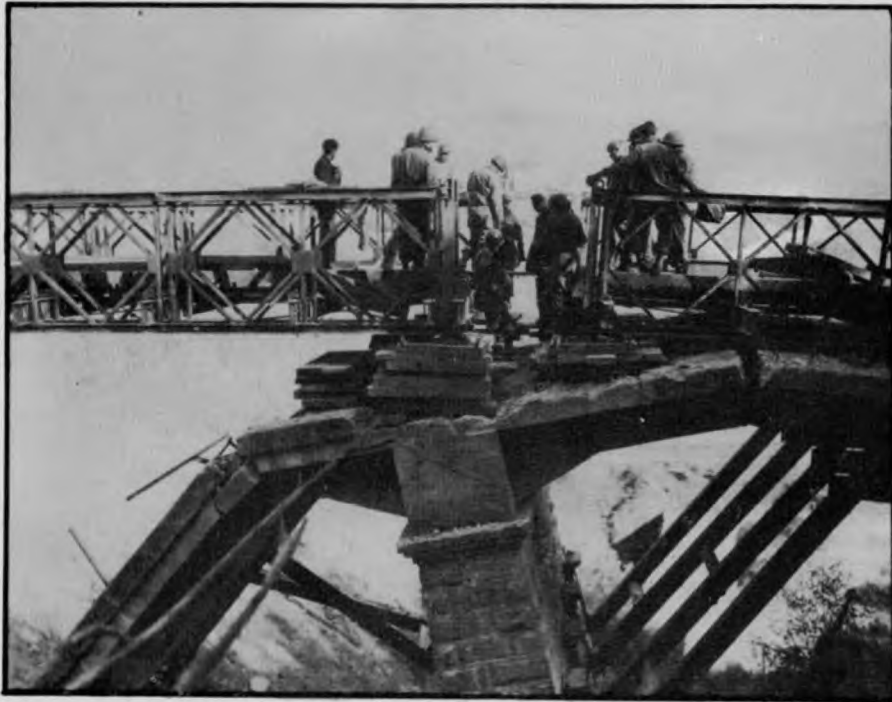
PIER HEAD WITH PACKING AND REINFORCEMENT
