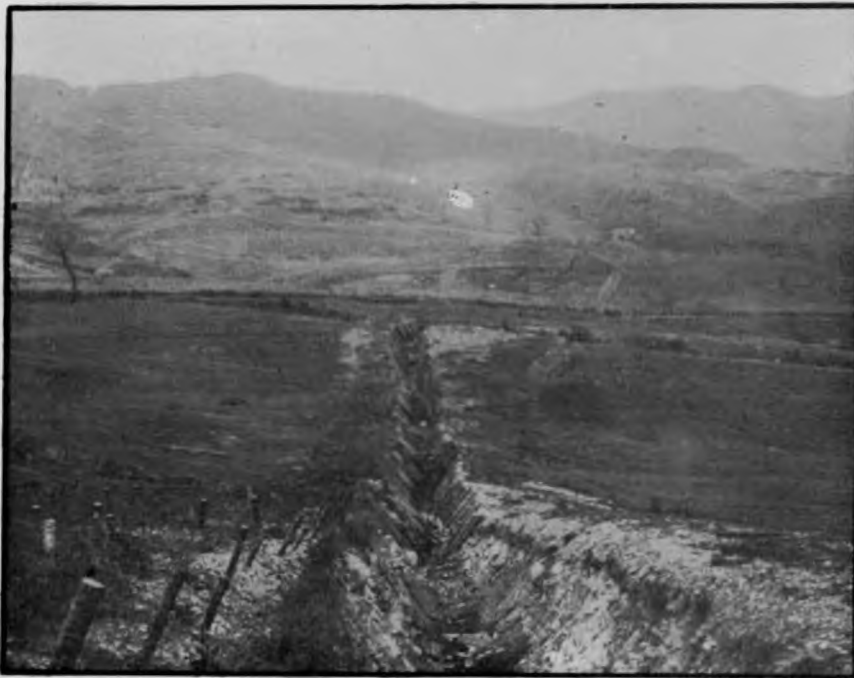
ANTI-TANK DITCH, WIRE ENTANGLEMENTS AND CONCRETE PILLBOX IN FUTA PASS DEFENCES
