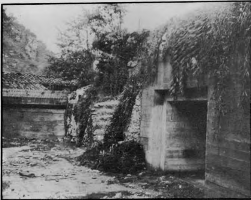
GERMAN CONCRETE PILLBOX AND ANTI-TANK WALL (LEFT)
