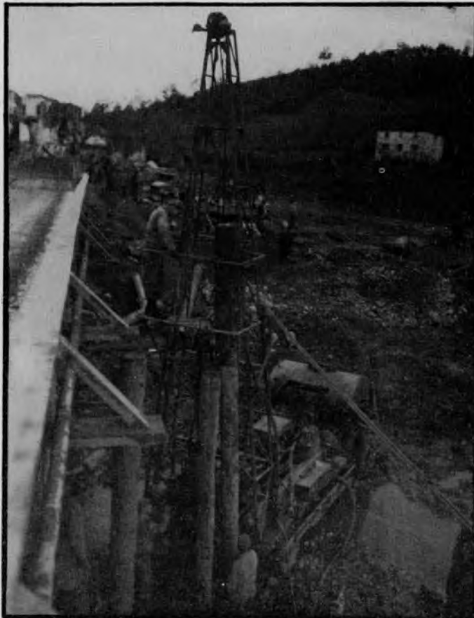
ROTARY: SETTING PILE
