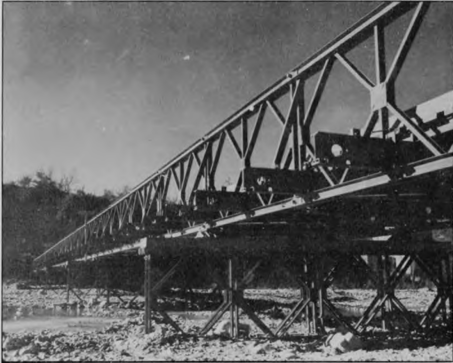
PIERS SET AT 40 ft.
