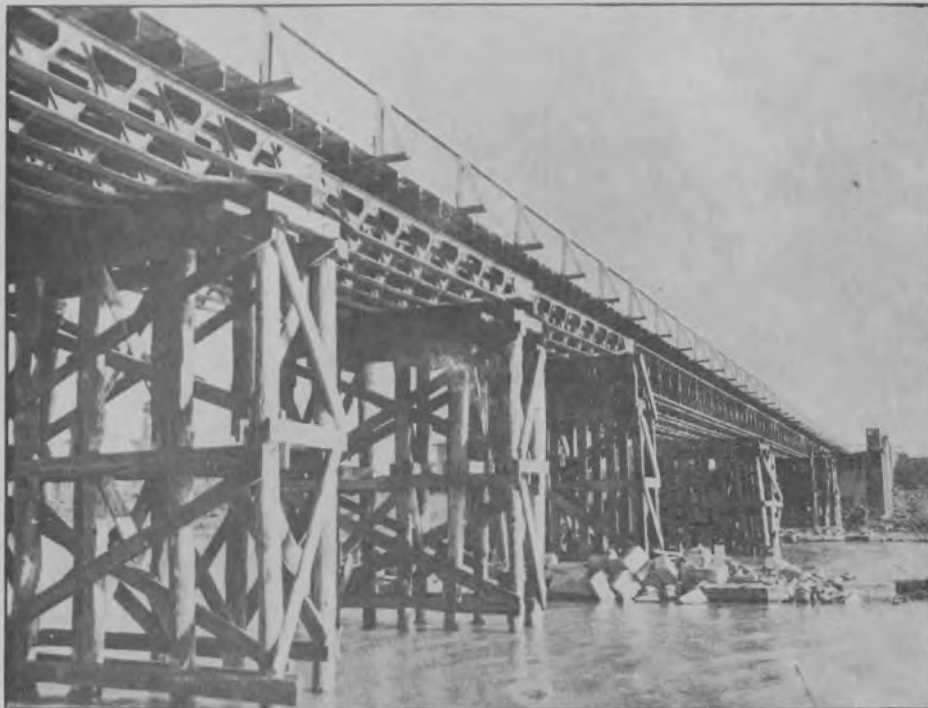
CLOSE UP OF COMPLETED BRIDGE
