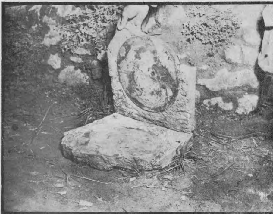
OPEN VIEW OF TELLERMINE EMBEDDED IN CONCRETE
