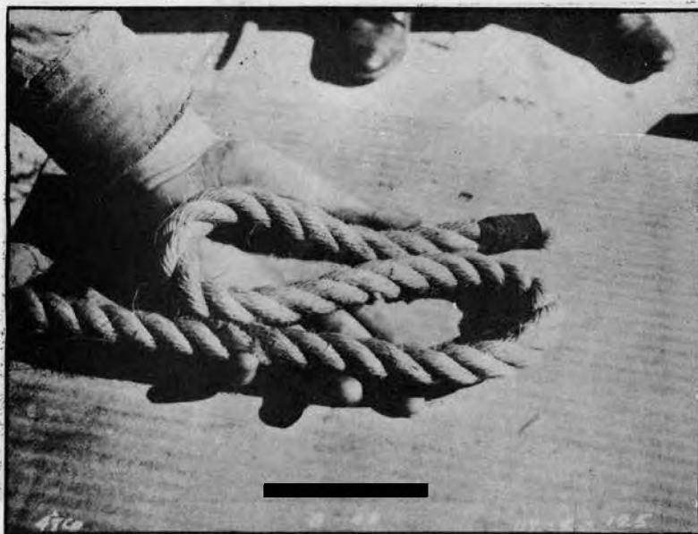
FIG. 12. Second step in preparing a cats paw.
