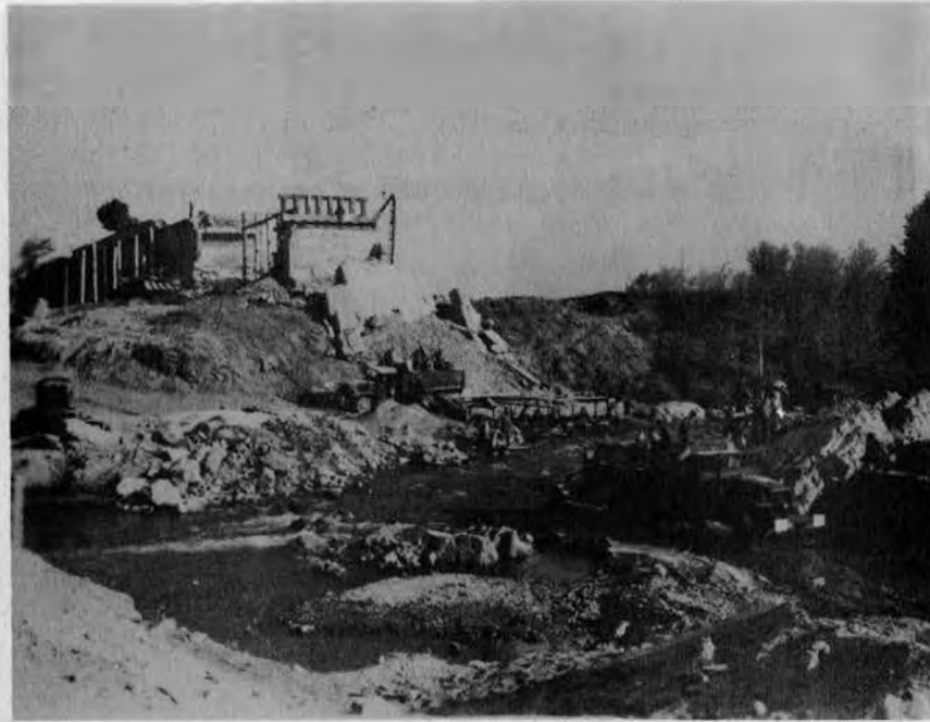
BEGINNING OF CONSTRUCTION SHOWING DEMOLISHED BRIDGE
