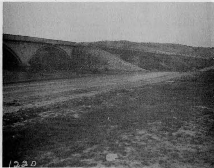
COMPLETED BRIDGE NORTH VIEW
