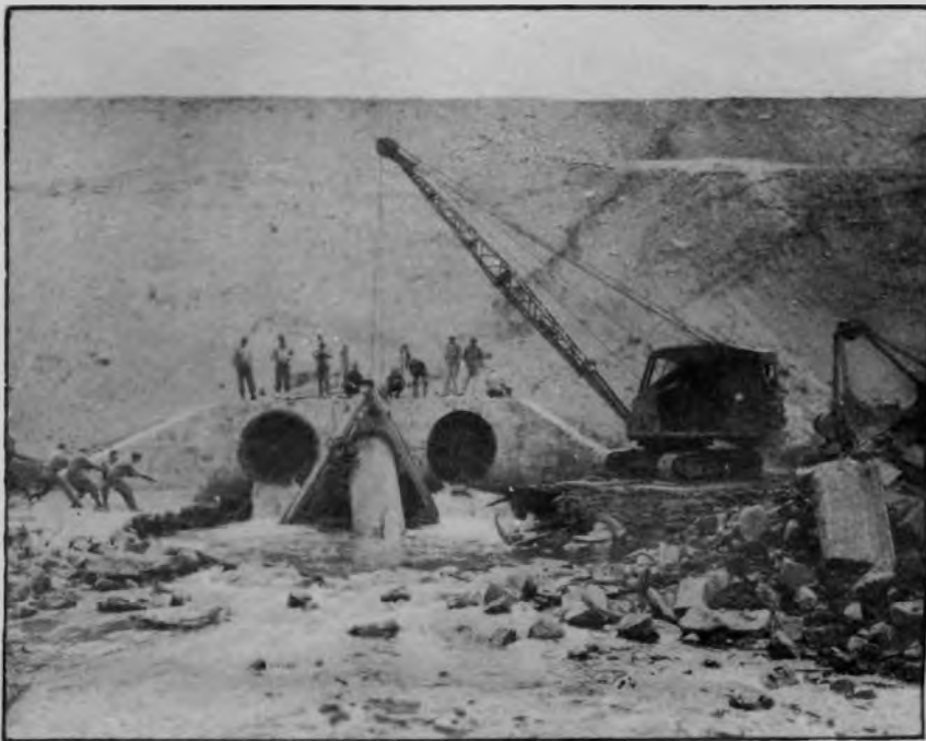
Figure 6 Placing of Outlet Section and A-Frame.
