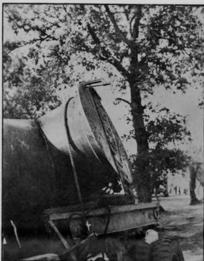
Figure 4 Gate on Outlet end of Siphon before Installation.
