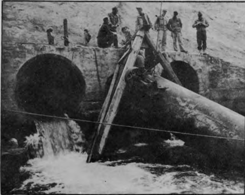
Figure 5 Placing of Outlet Section and Supporting A-Frame Showing Gate-opening Winch.
