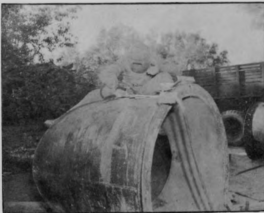
Figure 3 Fabrication of Bent Section of Siphon by Arcwelding.
