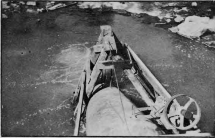
Figure 9 View of Outlet Section with Siphon in Operation
