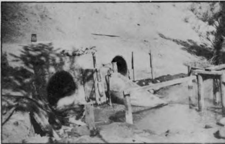
Figure 10 View of Inlet Section with Siphon in Operation Water level in Pool Lowered about one foot.
