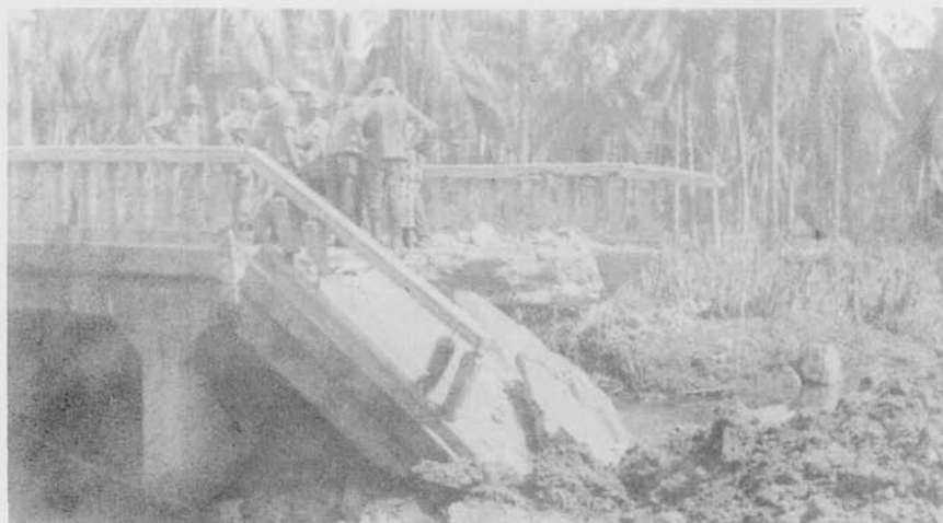
Result of Jap demolition of Bridge over BALIWASAN River, looking northwest. Repairs were effected by dumping river gravel to fill the break and using remaining span to carry the river flow.
