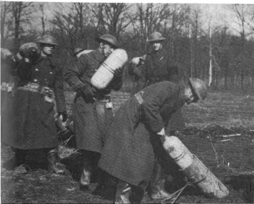
LOAD! Installing gas cylinders in Livens projectors.
